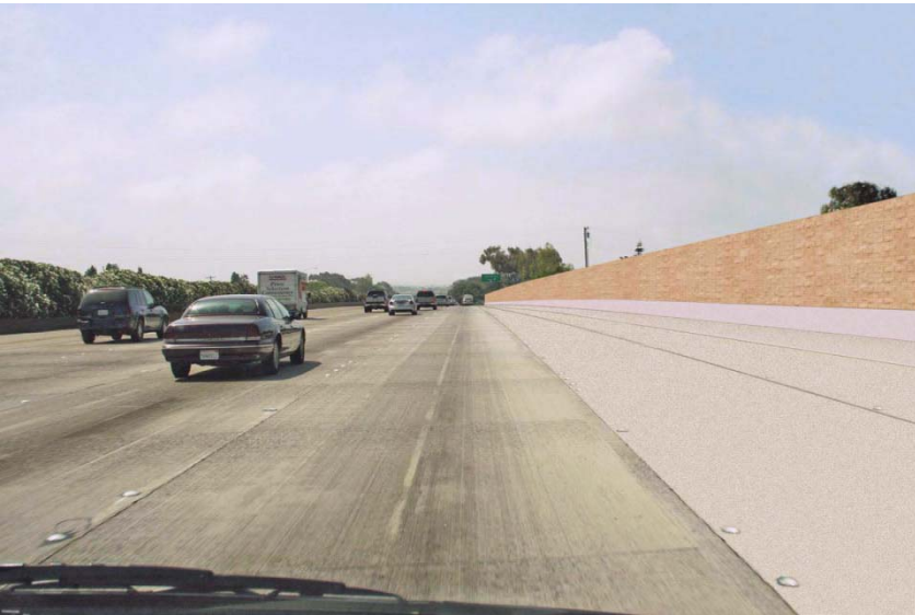
TAMARACK AVE SB I5 AFTER
