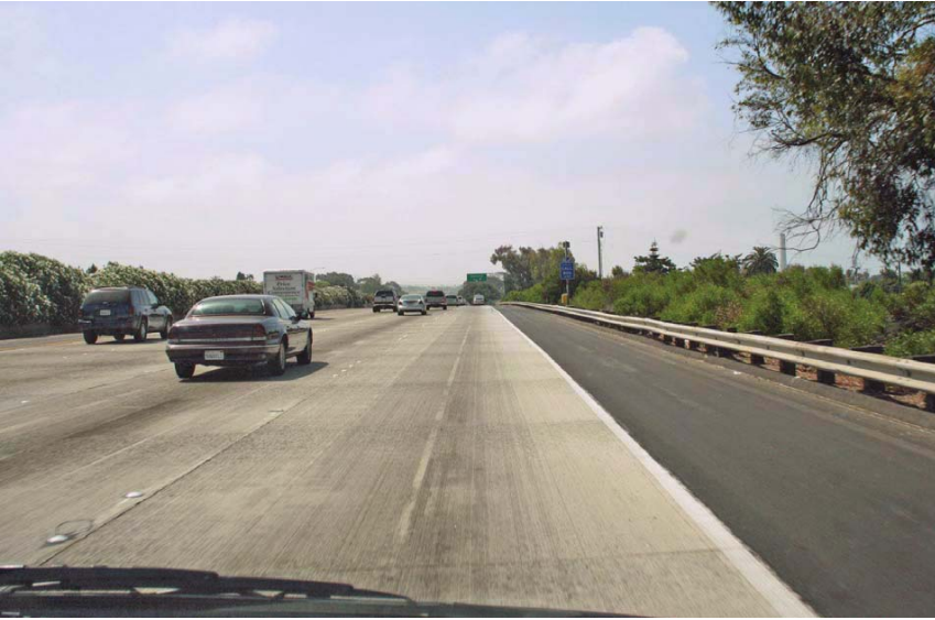
TAMARACK AVE I5 SB BEFORE
